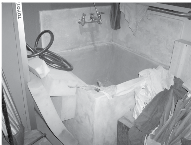
Jody Thomas had a water pit installed that self-drains. Photo by the author.
