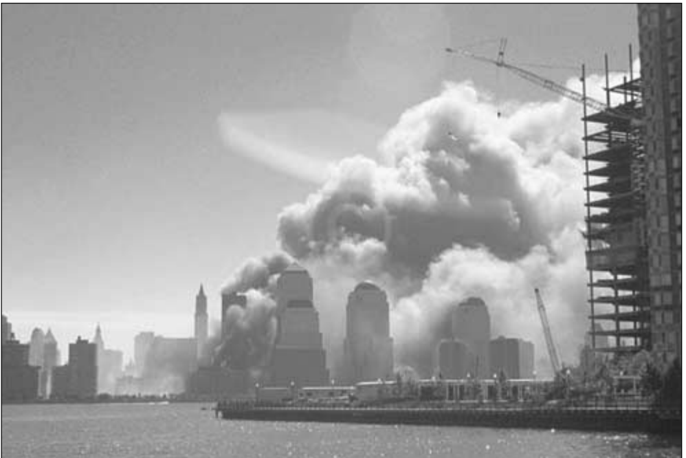
FIGURE 12.1 The September 11, 2001 terrorist attacks on the World Trade Center created a new imperative on the issues of building security.
