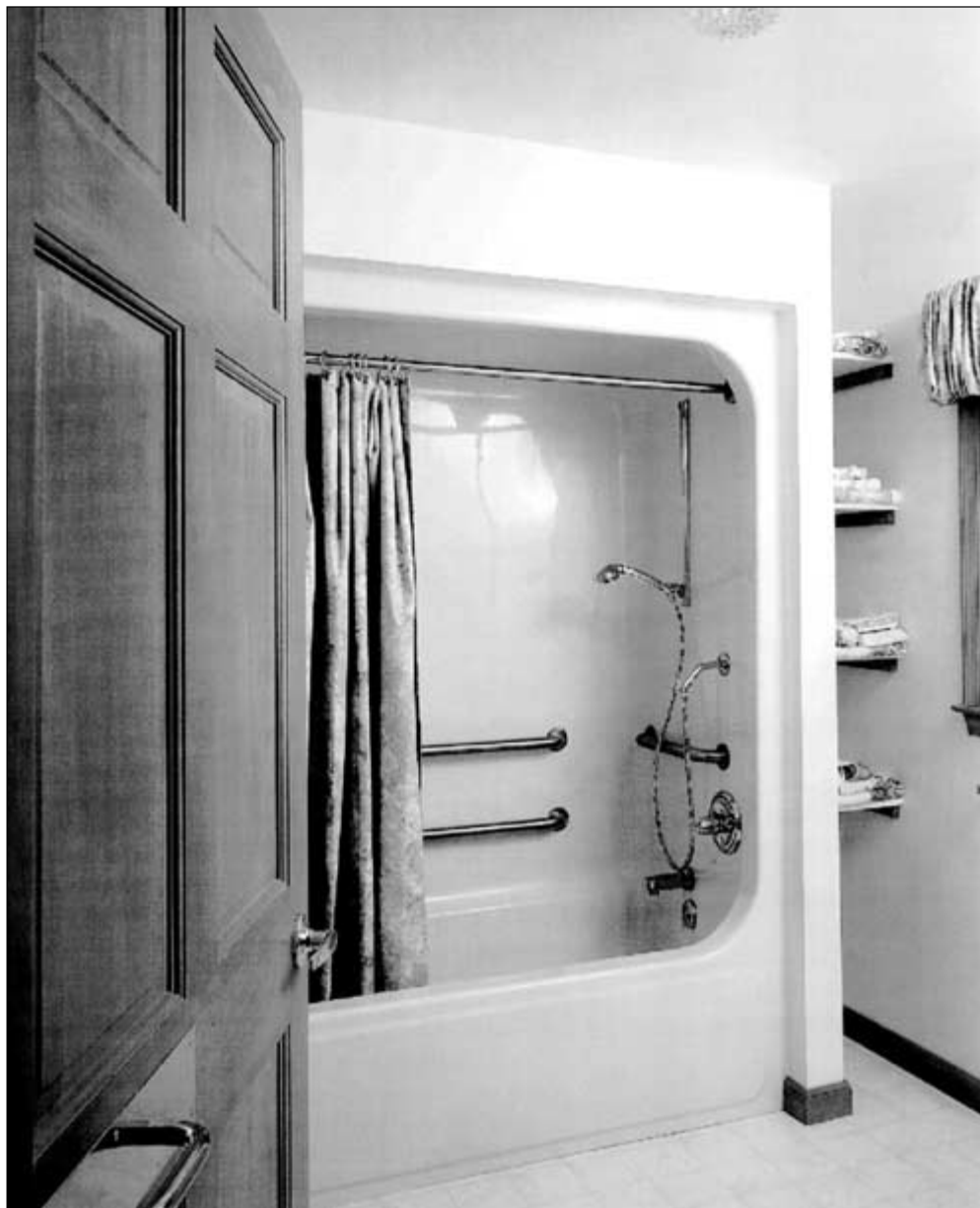
FIGURE 9.21 Prefabricated shower unit with strong grab bars. (Courtesy Charles A. Riley II, High-Access Home , Rizzoli International Publications, Inc.)
