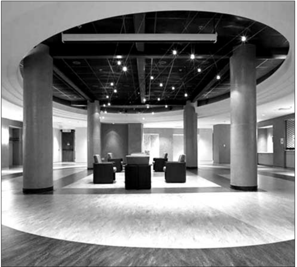
FIGURE 5.10 The use of cold cathode lighting in a municipal building in Toronto, Ontario. (Courtesy Cathode Lighting Systems Inc., Maryland)
