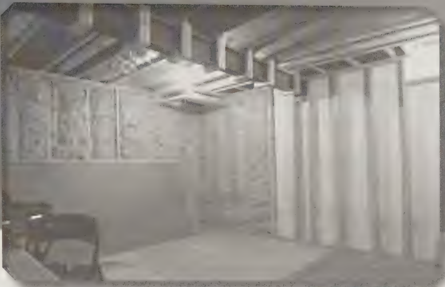
Adding the Insulation in the Walls
