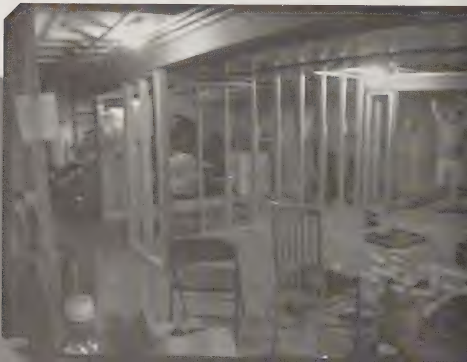
Framing the Walls of a Studio
