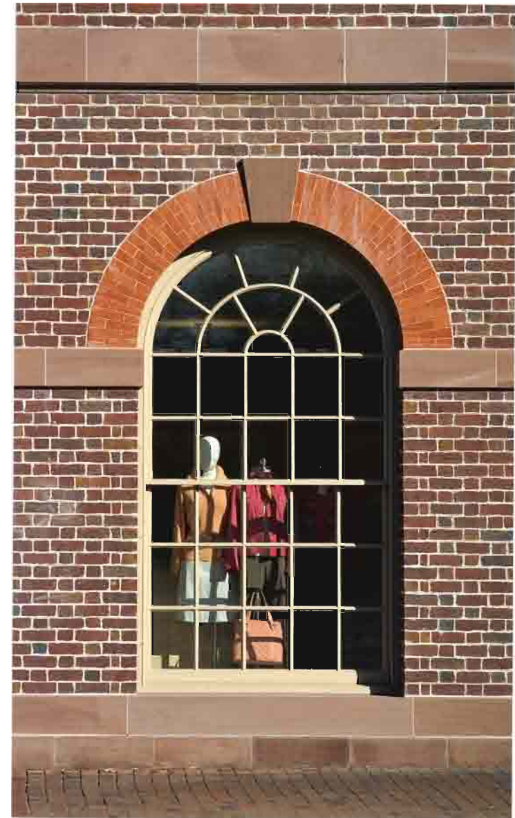
Detail of arched window of Corner building, showing color combination of local field brick, English rubbed and gauged brick arch with St. Bees sandstone, plinth, impost, and string course
