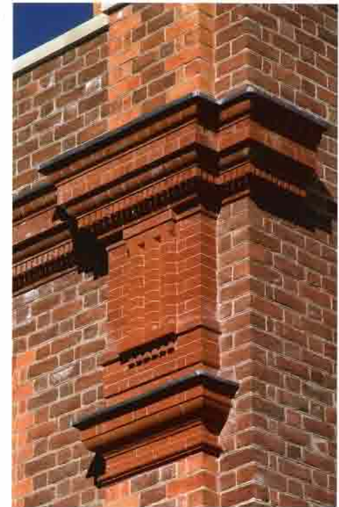
Detail of rubbed and gauged Doric entablature to the Northwest building
