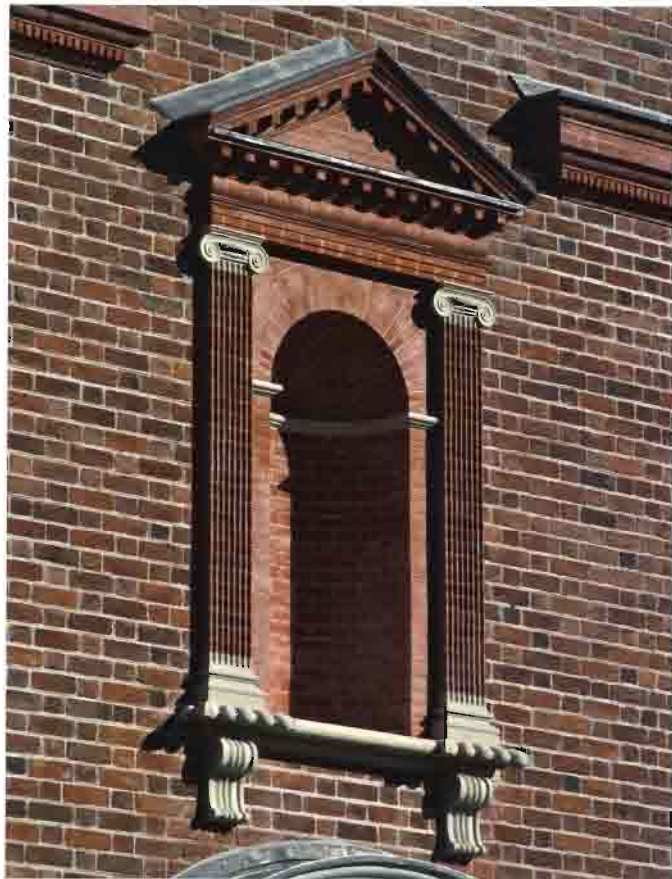
BOTTOM Niche to the center of the Northwest building showing rubbed and gauged fluted pilasters, pediment, and niche with Ionic capitals, bases, gradoons, and consoles in Portland stone
