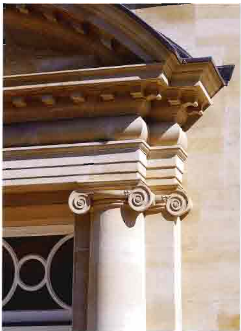
Detail of Ionic capital and pediment to entrance door on south front
