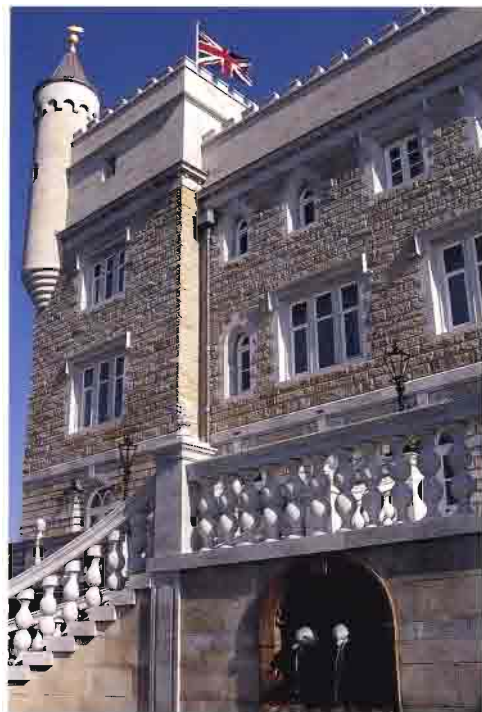
Detail of north front
