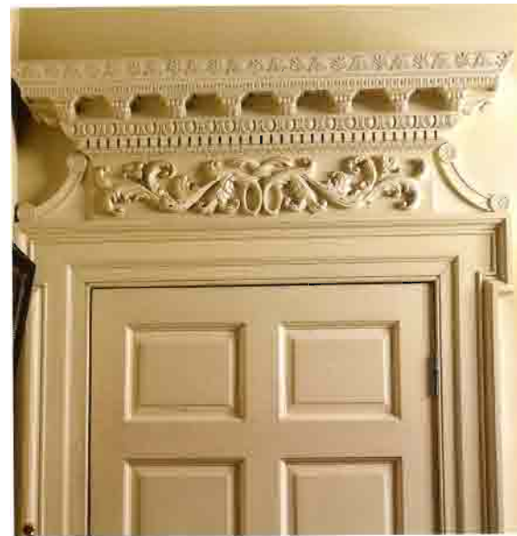
ABOVE White Room, doorcase
