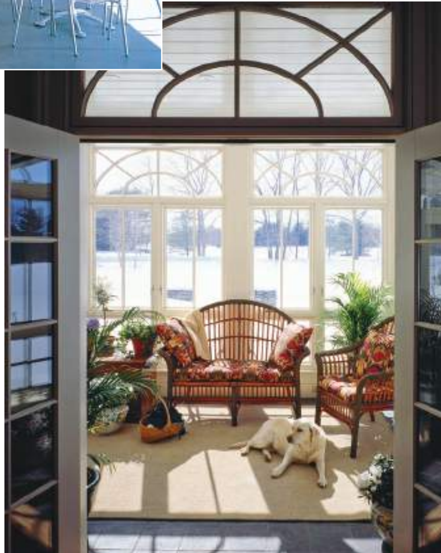
Figure 7.27 Passive solar heating is gained in this attached solarium. The French doors are opened to bring natural solar-heated air into the home during cloudless days, even in the deepest of wintertime. The French doors are closed at night and on cloudy days when the solarium is chilly to keep the gained heat in the interior living areas. Design by Whitten Architects/photo © Brian Vanden Brink
