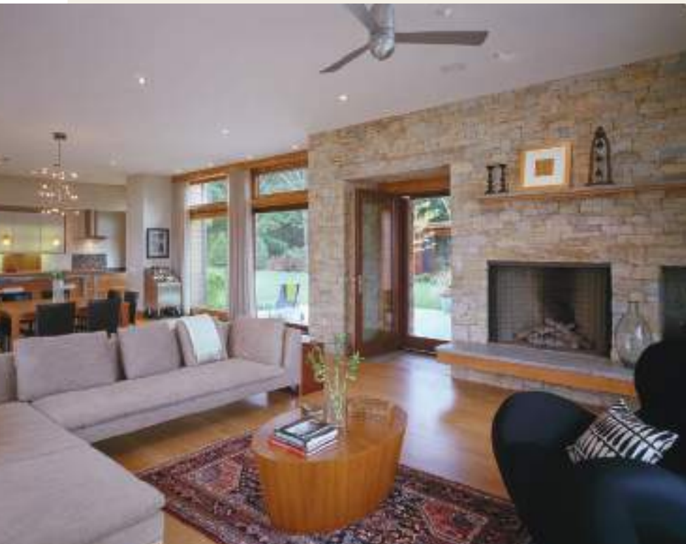
Figure 11.2 A natural stone in ashlar configuration frames this fireplace and French door. Stone is a durable, timelessly handsome wall treatment that requires little to no maintenance. Design by Hutker Architects/photo © Brian Vanden Brink
