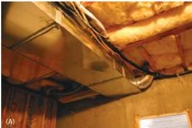
Figure 7.23 (A) Ducts or ductwork is the system that brings heated air from a furnace to all areas of the home. This shows ductwork in an unfinished basement and insulation in the floorboards, to be covered later with Sheetrock when the basement is finished. The smaller duct leads to a register in the floor. Rough electrical wiring is also seen here. (B) This central air-conditioning unit provides refrigerated air to the home. These units are efficient, but generally costly to run in terms of electricity used. Photo © Kathryn Taylor
