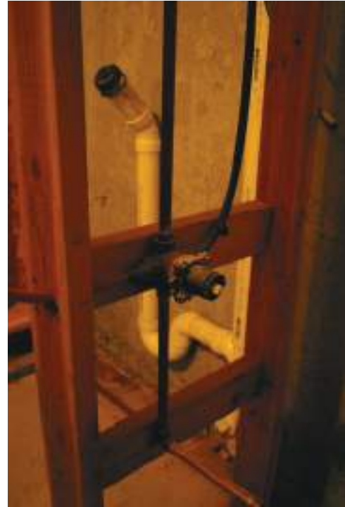
Figure 7.19 Rough plumbing is installed after the wall is framed. The black and copper pipes will carry fresh, culinary water to sinks, dishwashers, bathtubs, showers, and washing machines. The larger white pipe will carry away the waste water. Photo © Kathryn Taylor
