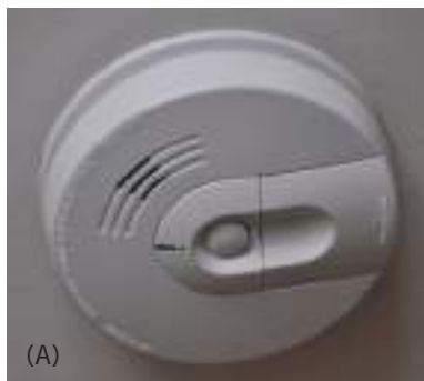
Figure 5.30 Typical residential electronic devices include (A) a smoke detector and (B) intercom. Photos © Kathryn Taylor
