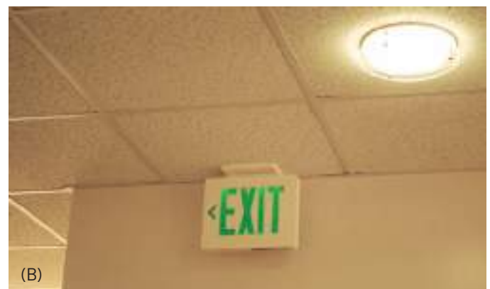
Figure 7.30 (A) The plenum is the area above the ceiling; here a suspended ceiling of acoustical tiles provides access to any of the systems in the plenum, including the lighting, heating/ventilation/air-conditioning (HVAC), the projection system, or the fire alert/sprinkling system. (B) Egress lighting must be visible both when the lighting works and when there is a temporary electrical outage or emergency, in which case the LED lights continue to operate to lead users to outdoor safety. Photo © Kathryn Taylor
