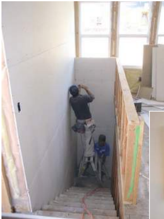
Figure 7.17 Sheetrock may be finished as rough plaster, as lightly textured, or with a smooth finish. Here installers attach drywall panels with screws. The seams will be covered with plaster (mud) and tape, and the screw holes will also be filled with plaster. Photo © David A. Taylor
