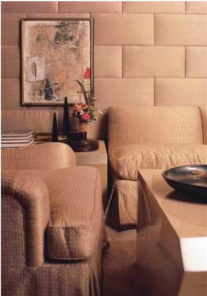
Figure 11.12 Fabric on the wall, here wrapped as blocks or upholstered, absorbs noise and increases comfort. Courtesy of DuPont “Teflon” soil and stain repellent
